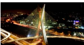
Brazil Infrastructure Paving the Way May 5, 2010
